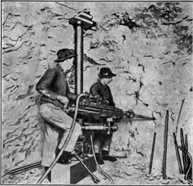
Fig. 24. Chicago Giant Rock Drill on Column Mounting — Tunnel Work.
